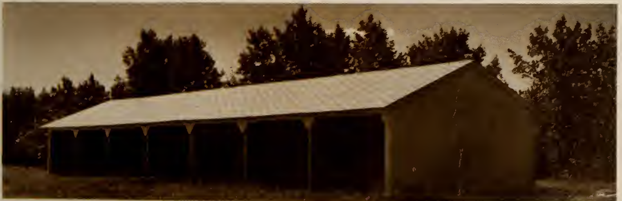
Pole Shed - This is a clear span pole shed building. It will be used for winter shelter.
