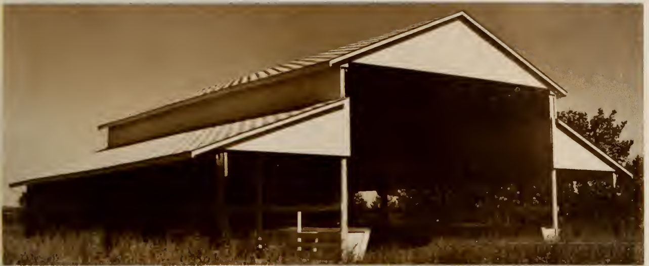
Hay Shed Feeder - Central portion is the hay storage feeding into covered feed bunks on either side.
