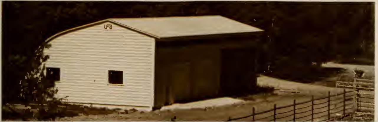
Half-Arch Building - This building lends itself particularly well to where a high front is needed to get equipment through. On the Charrouse Ranch, this building is used for a workshop, tractor, trailer garage, and covered storage.
